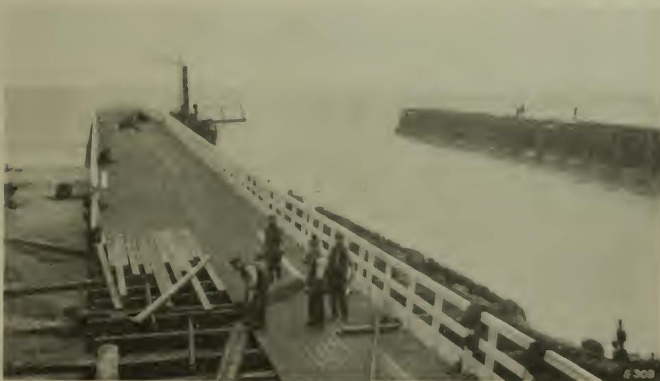
FIG. 5. THE QUAY IN COURSE OF CONSTRUCTION.
